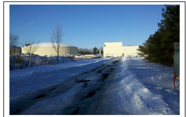
Processing Plant De-Icer Management System
